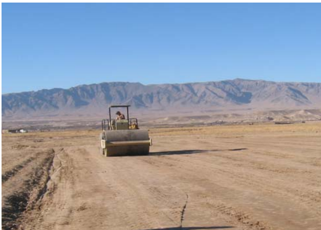
Compacting the treated runway
